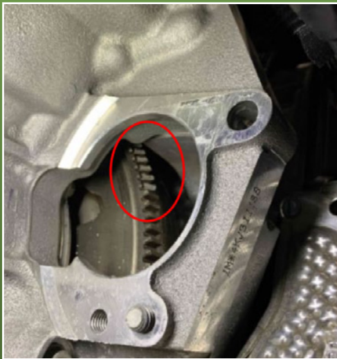
Check for damaged flex plate teeth through the starter mounting hole.
