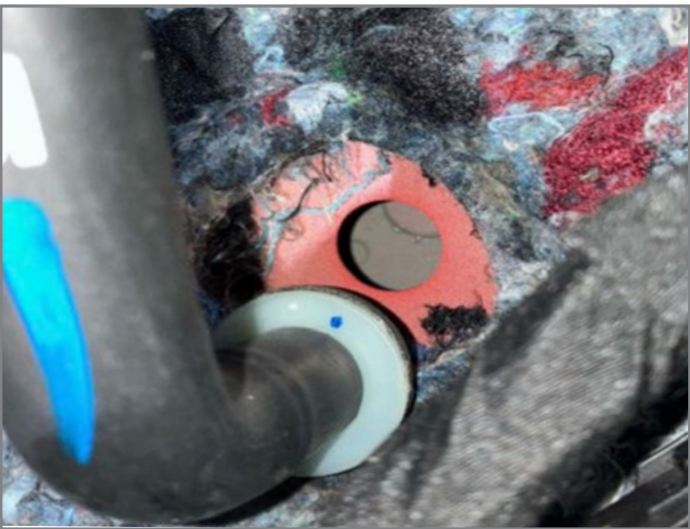
Disconnected drain tube
