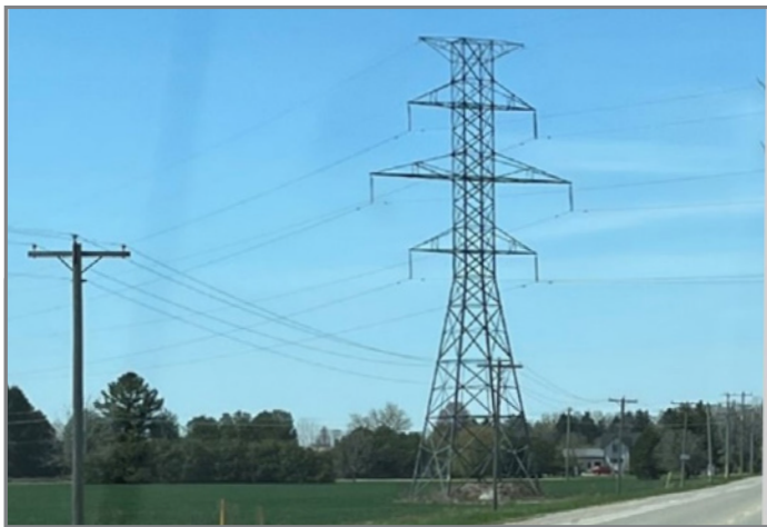
Aluminum roof bows of an upfitter box may act as an antenna when passing under high-voltage lines.
