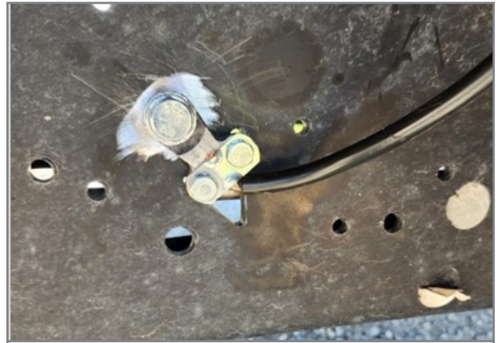
Ground cable attached to the vehicle frame
