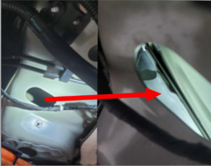
Body hole on the passenger's side of the frame
