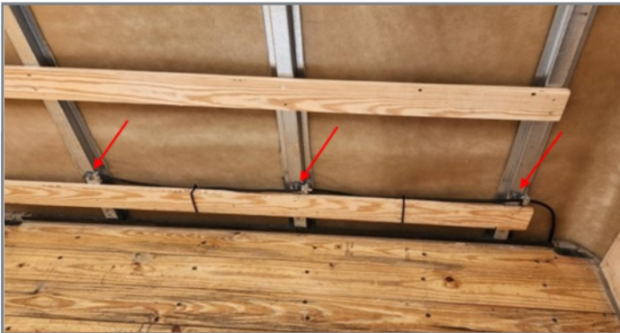
Ground cable installation across the first three roof bows.
