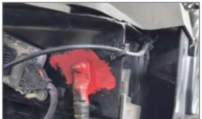
Check eyelet clamp load and red anti-corrosion paint
