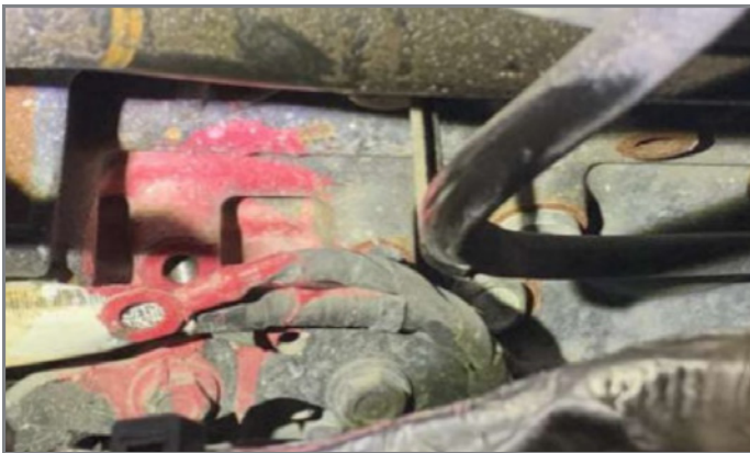
Red anti-corrosion paint.
