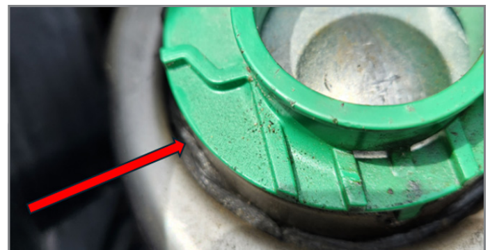
New polyethylene foam seal installed around filler opening.
